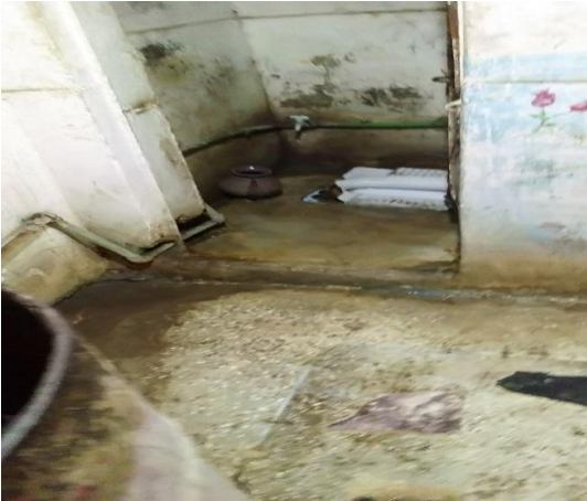
Inner condition of toilet room
