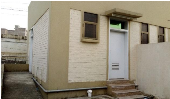
Public toilet constructed by MSP but not-functional
