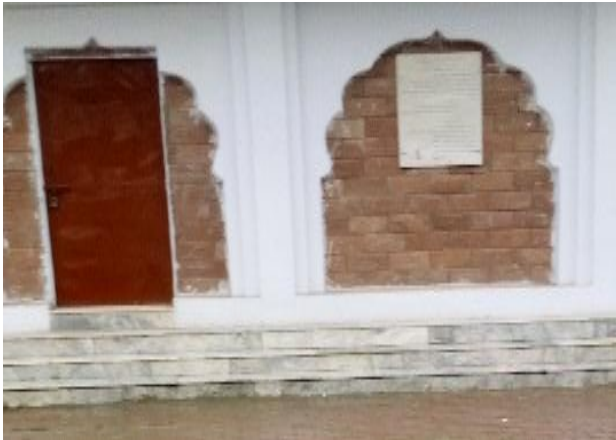
Closed toilet in Shalimar Garden
